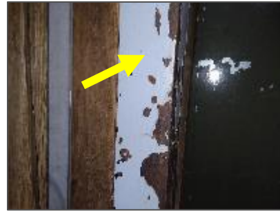
Photo 16: Grey paint on the metal door frame in the Animal Stalls.
