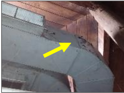
Photo 15: Grey paint on the metal duct in the Animal Stalls.
