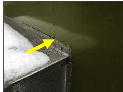
Photo 4: Non-asbestos grey / green mastic on an HVAC unit on the roof.
