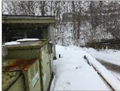
Photo 14: Non-asbestos roofing over the flat portion of the roof.
